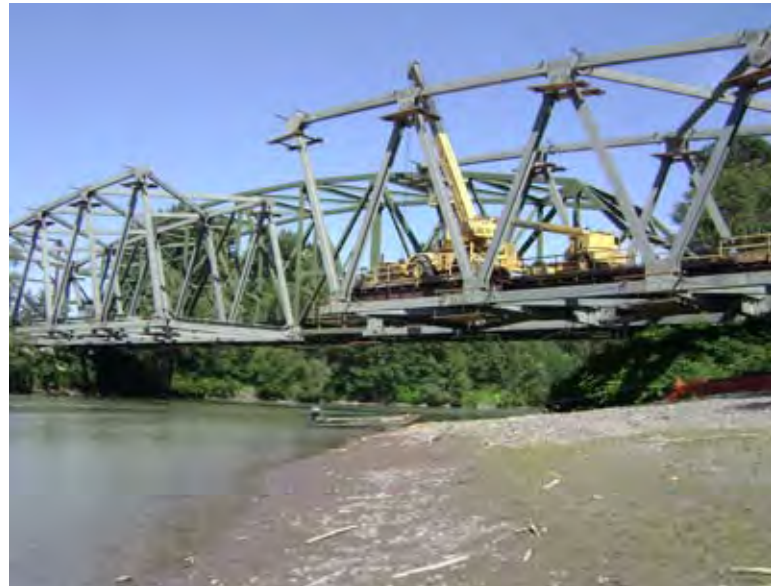
Because access for a large land-based crane was not available on the south shore of the Nooksack River crossing, the anchorage and backstay system had to support the weight of equipment as well as the truss weight.
