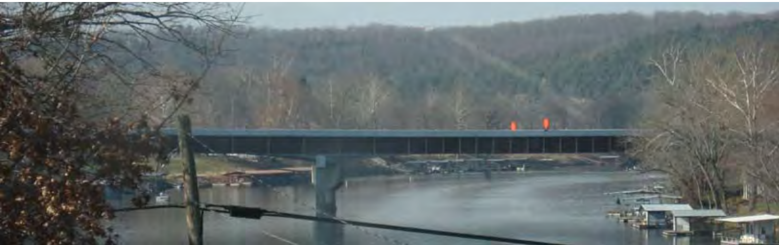
Above: The two main spans are 230 ft long, and the bents were skewed at 20° to match the river’s flow.
