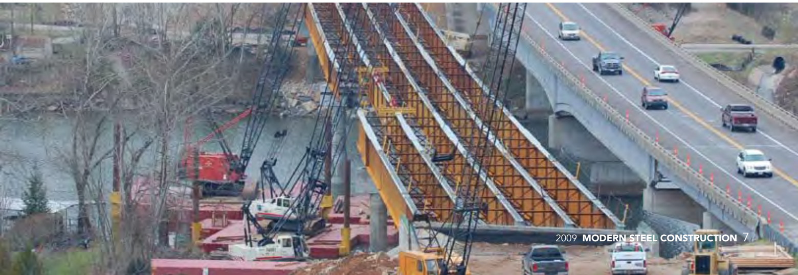
Above: The two main spans are 230 ft long, and the bents were skewed at 20° to match the river’s flow.
