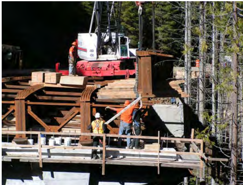
Below: Located along a remote and extremely windy stretch of Oregon highway, the Diamond Creek Bridge site required tight clearances to minimize environmental disturbance.
