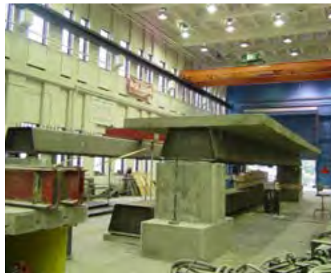
Fig. 4 With the concrete deck in place, several sections of a folded plate girder bridge can be stacked and shipped to the site on one trailer.
