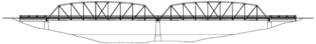
The original bridge built in 1921 had two 166-ft-long truss spans with short approach spans.
