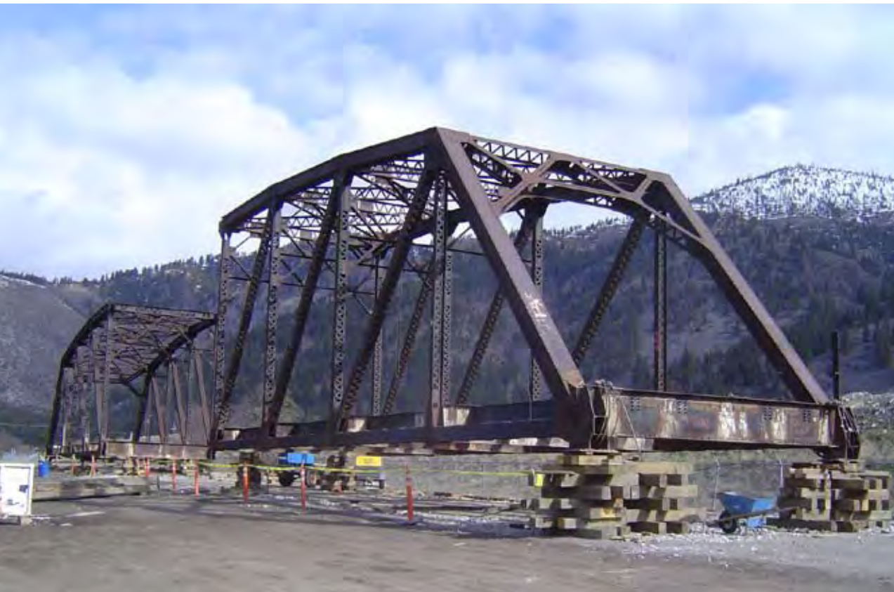
One old truss span was removed to the river bank for reconstruction, where it was split apart and new steel added to lengthen the span. Steel from the second truss span was used to replace damaged parts and steel stringers were used in the added truss bays.
