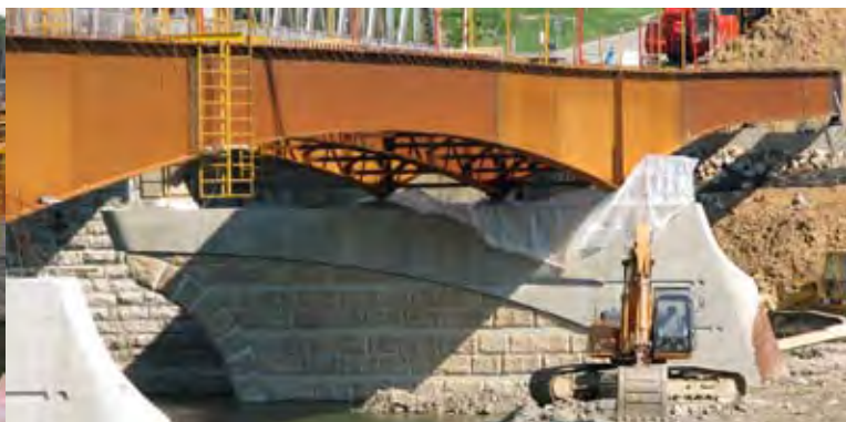
The welded plate girders range in depth from 6 ft at the center of the spans to close to 12 ft at the piers.
