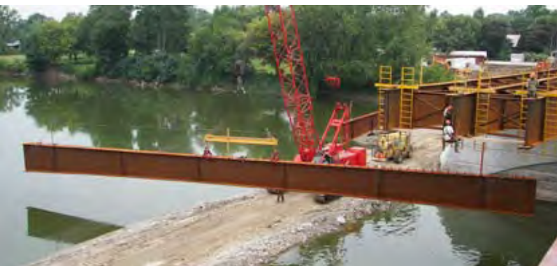
More than 800 tons of structural steel was used in the construction of the bridge.
