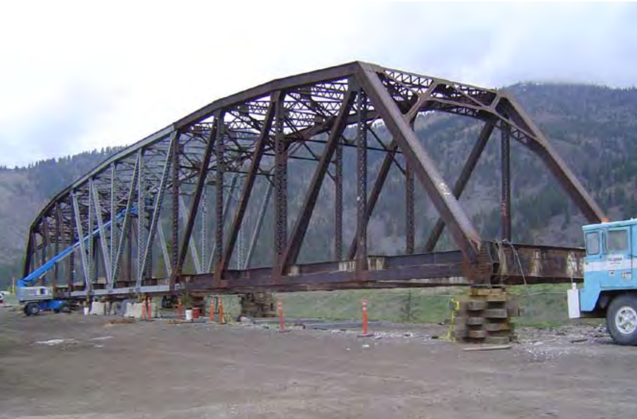
The old steel of the existing truss was cleaned by 5,000-psi water jetting with a roto-tip nozzle. Cleaning water and paint debris were collected, filtered and recycled. The reconstructed truss, along with the new approach spans, were painted semi-gloss black using a three-coat moisture cure urethane paint system supplied by Wasser.
